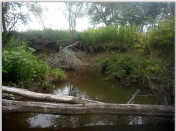
Figure 2.4: Neuman Creek Bank Erosion (BNR)
